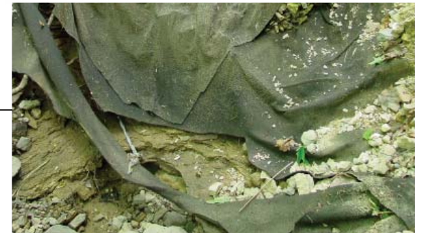
Ravine at Raymer's Cove — Deteriorating Outfall Due to Excessive Volume and Velocity of Storm Runoff
