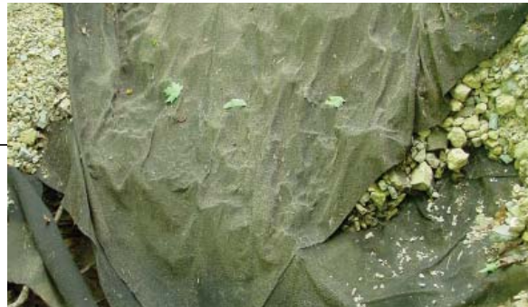
Ravine at Raymer's Cove — Deteriorating Outfall Due to Excessive Volume and Velocity of Storm Runoff
