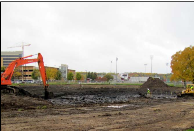
Stormwater pond takes shape north of lot 60.
