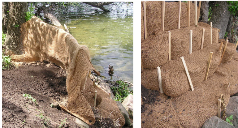
Figure 51. Photos of Soil Lifts in Progress and Completed (Prior to Planting) (photo by Rebecca Kagle).
