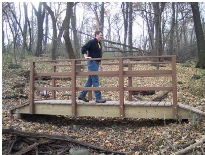
Figure 24. Muir Woods Footbridge (photo by Lars Higdon).
