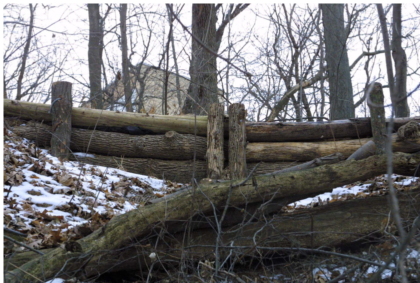
Figure 25. Log Retaining Wall (photo by Rebecca Kagle).
